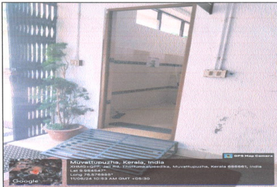
Ramp in front of wash room at ground floor (214)
