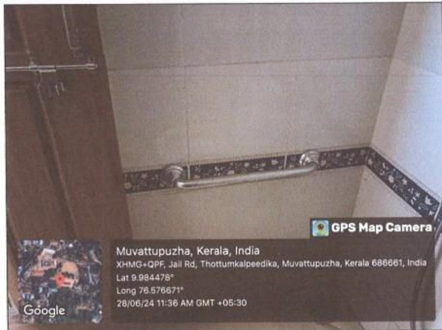
Handrail in the common washroom at the ground floor (214)
