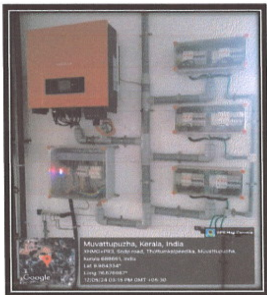
Solar Energy Control Panel
