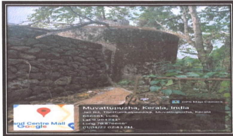
Rain Water Harvesting System to Prevent Wastage of Water
