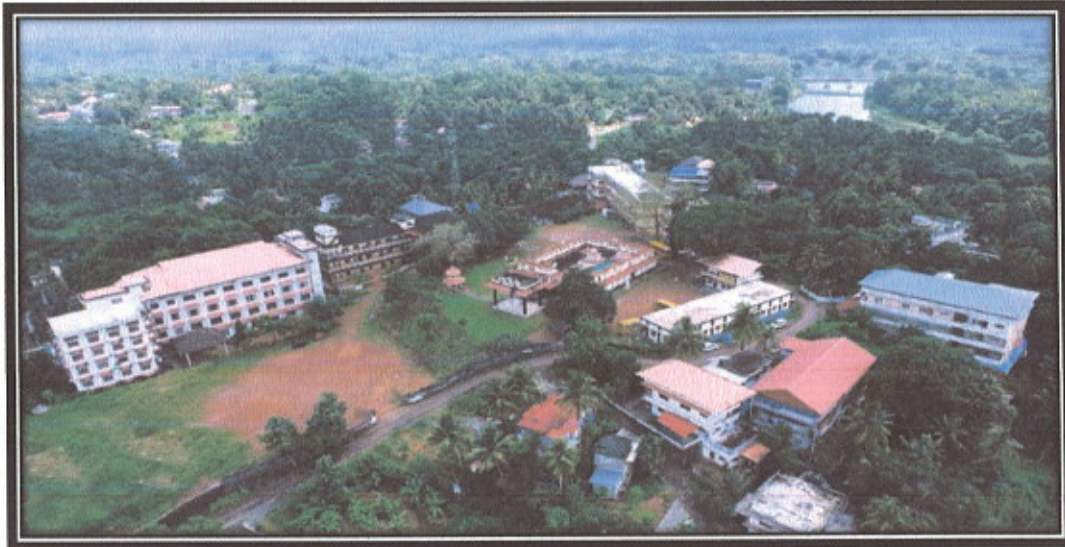
Clean Campus and its Surroundings; an Ariel View
