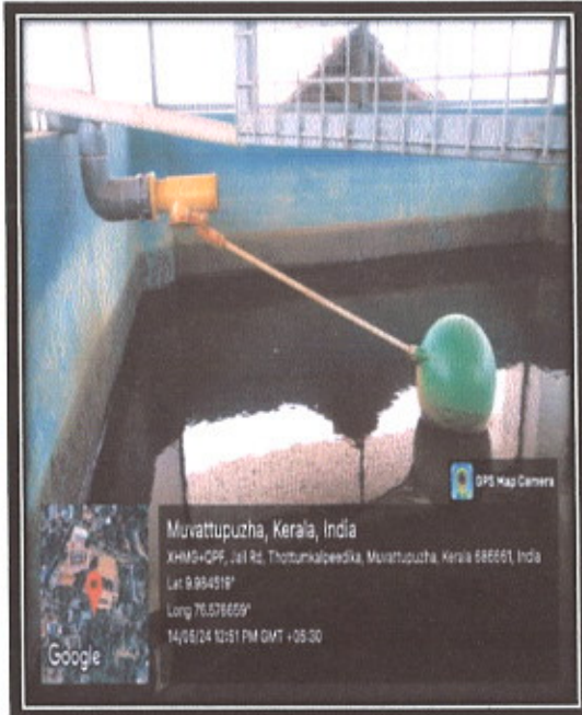
Ball Valve System to Prevent Overflowing
